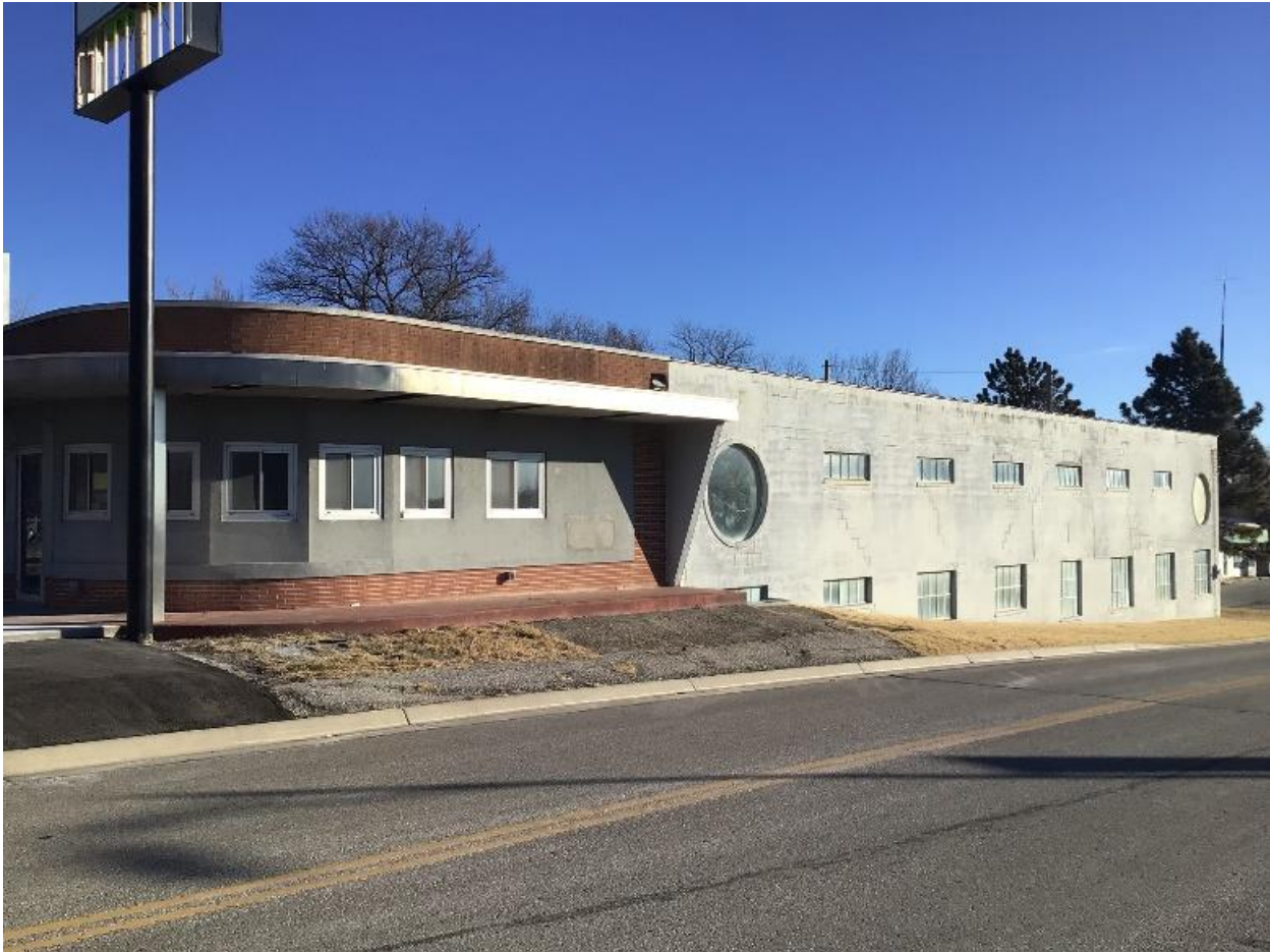
Photograph 16: 400 E 23rd Street
