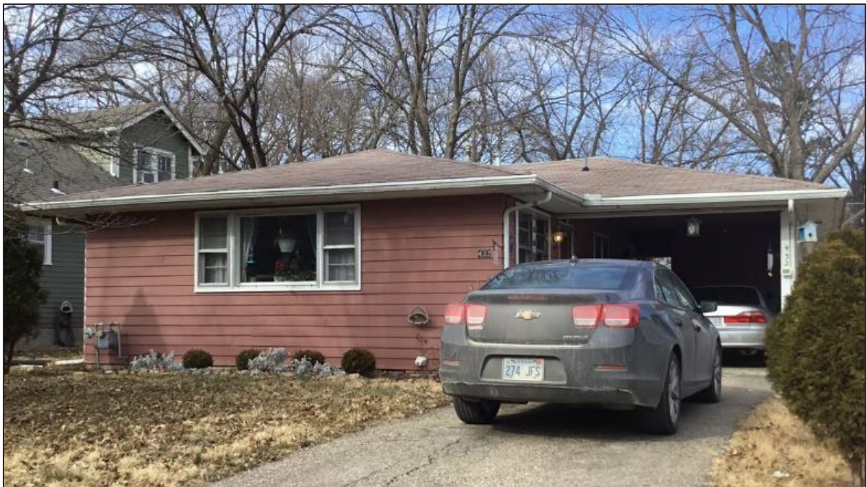
Photograph 24: 432 Forrest (ca. 1950; cross-hipped)
