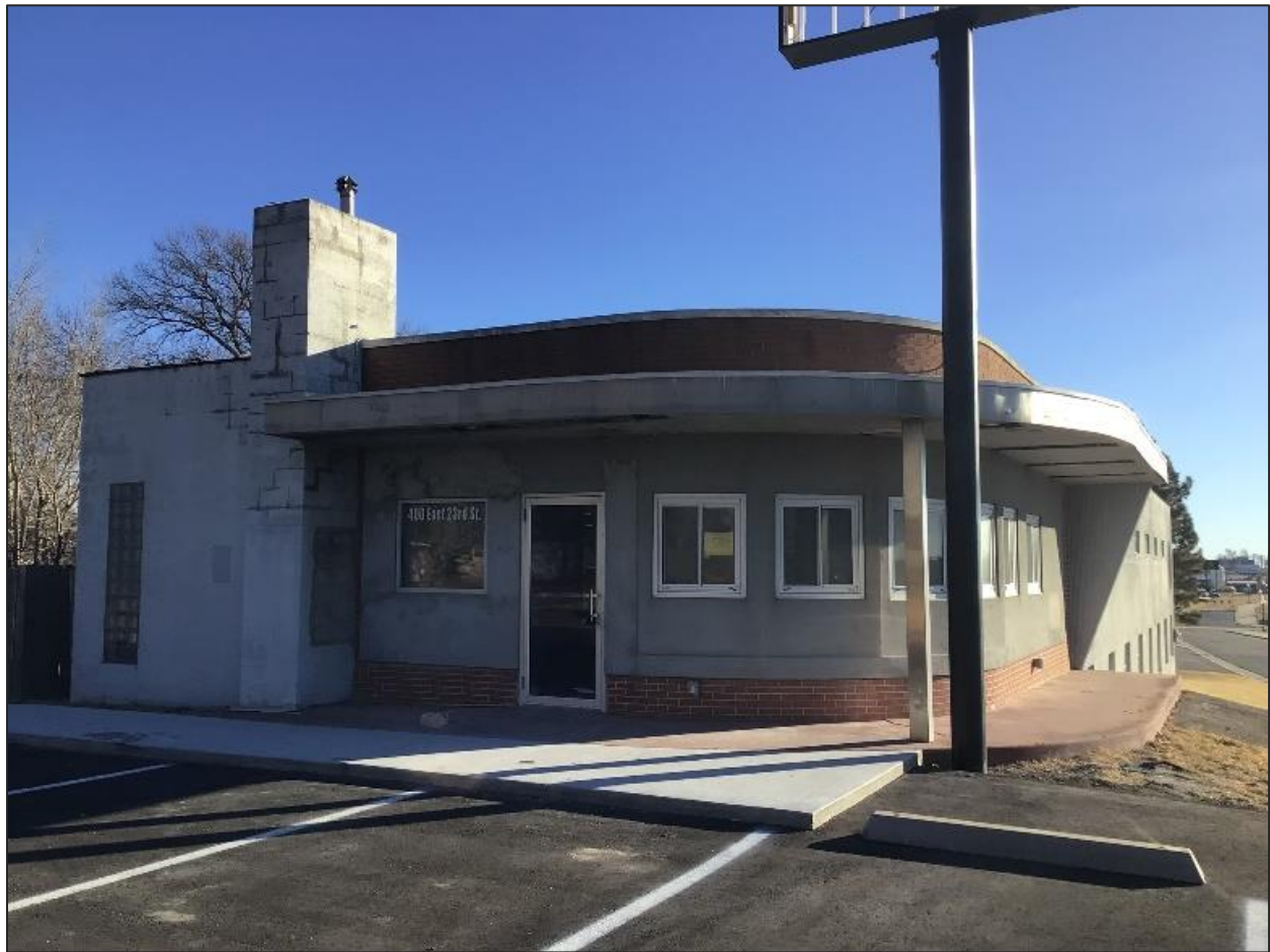
Photograph 17: 400 E 23rd Street
