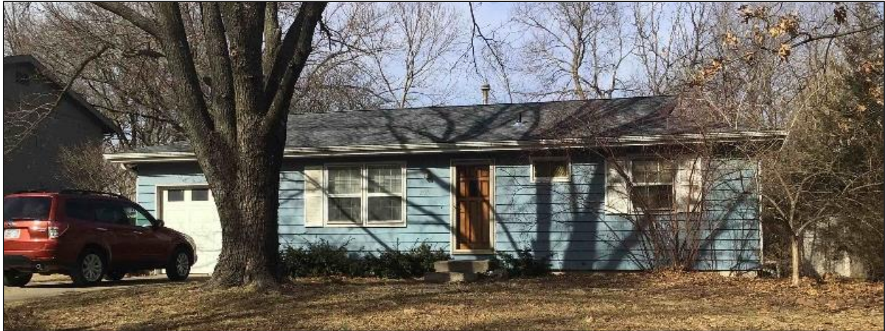
Photograph 25: 306 E 15th Place (ca. 1960; Ranchette/Minimal Ranch hipped roof)
