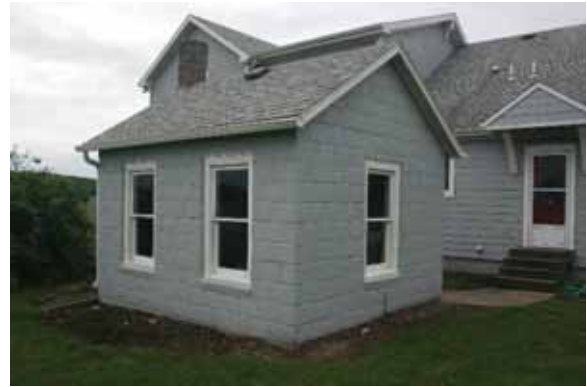
Electric Generating Building
