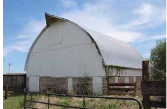
Gaines, Arthur, Barn
