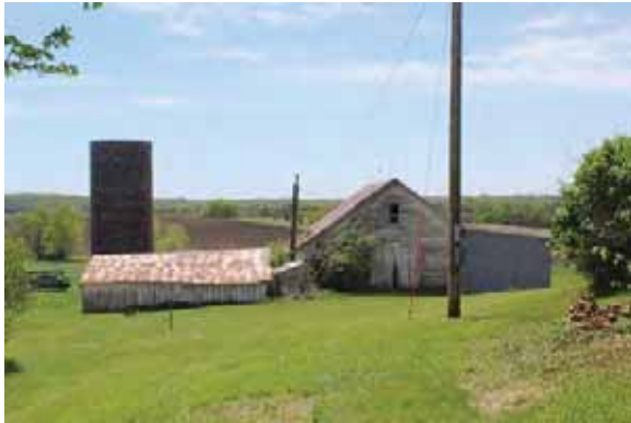
Barn 2 and Outbuildings
