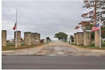
Marysville Cemetery Chapel. 1410 N. 16th Street. Looking east inside main entrance. 10/25/2023. Spencer Preservation/Spencer, Brenda.
