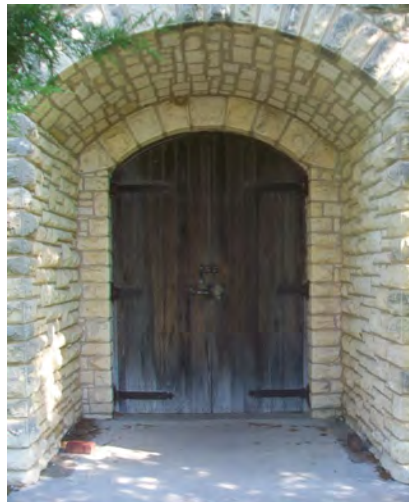
Marysville Cemetery Chapel. Marysville, Marshall County, Kansas. South Elevation Entrance. Photo by William E. Fischer, Jr., 9/1/2014
