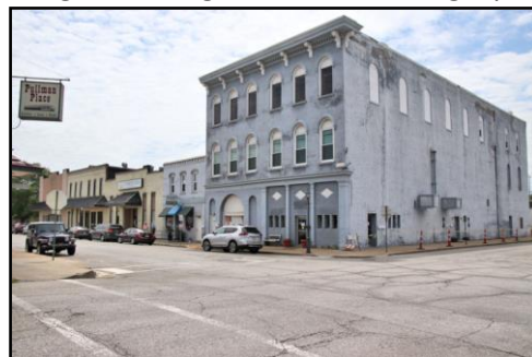
South side of the 200 block of Cherokee Street with the Stevens-Garrigue Iron Company Building on corner.
