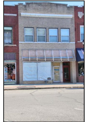
ca.1910s facade on 1880s building at 408 Delaware.
