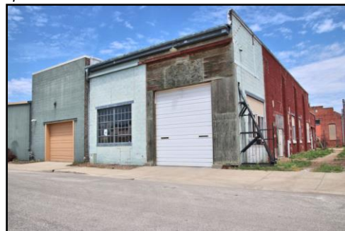
Two mid-century Warehouse buildings at 224-226 Choctaw.
