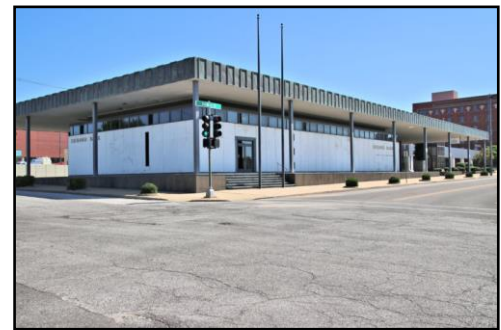
First National Bank Building at 630 Delaware (1965)
