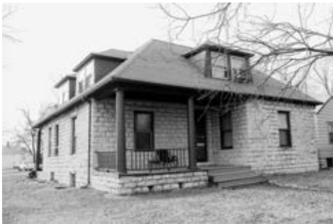
501 Pierre Street Vernacular Stone House with a Pyramidal Roof (also known as an Equilateral Hipped Roof)
