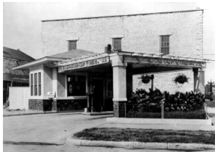
Houston and 3 rd Streets photograph courtesy of the Kansas State Historical Society
