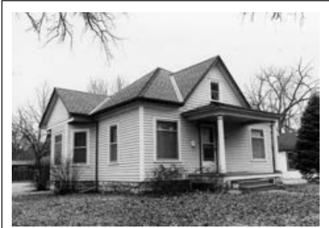
530 Moro Street Turn of the Twentieth Century Vernacular Folk House
