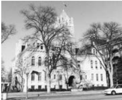
Riley County Courthouse Romanesque Revival Style
