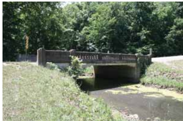
Lone Star Park Bridge No. 2
