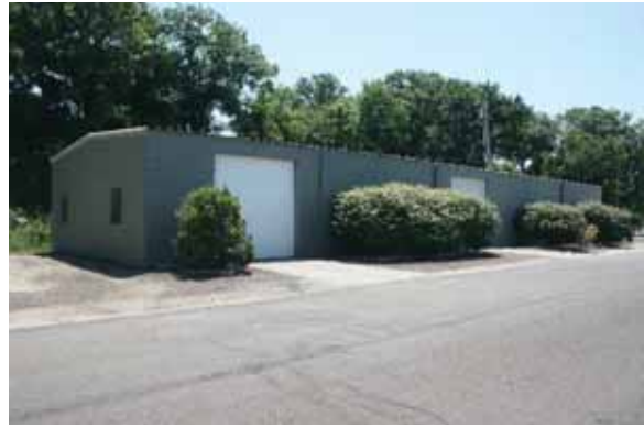
Maintenance Building – 1966 est.
