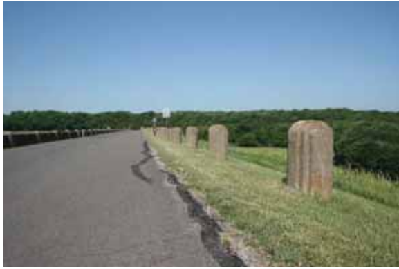
Concrete Pylons – North Side of Dam
