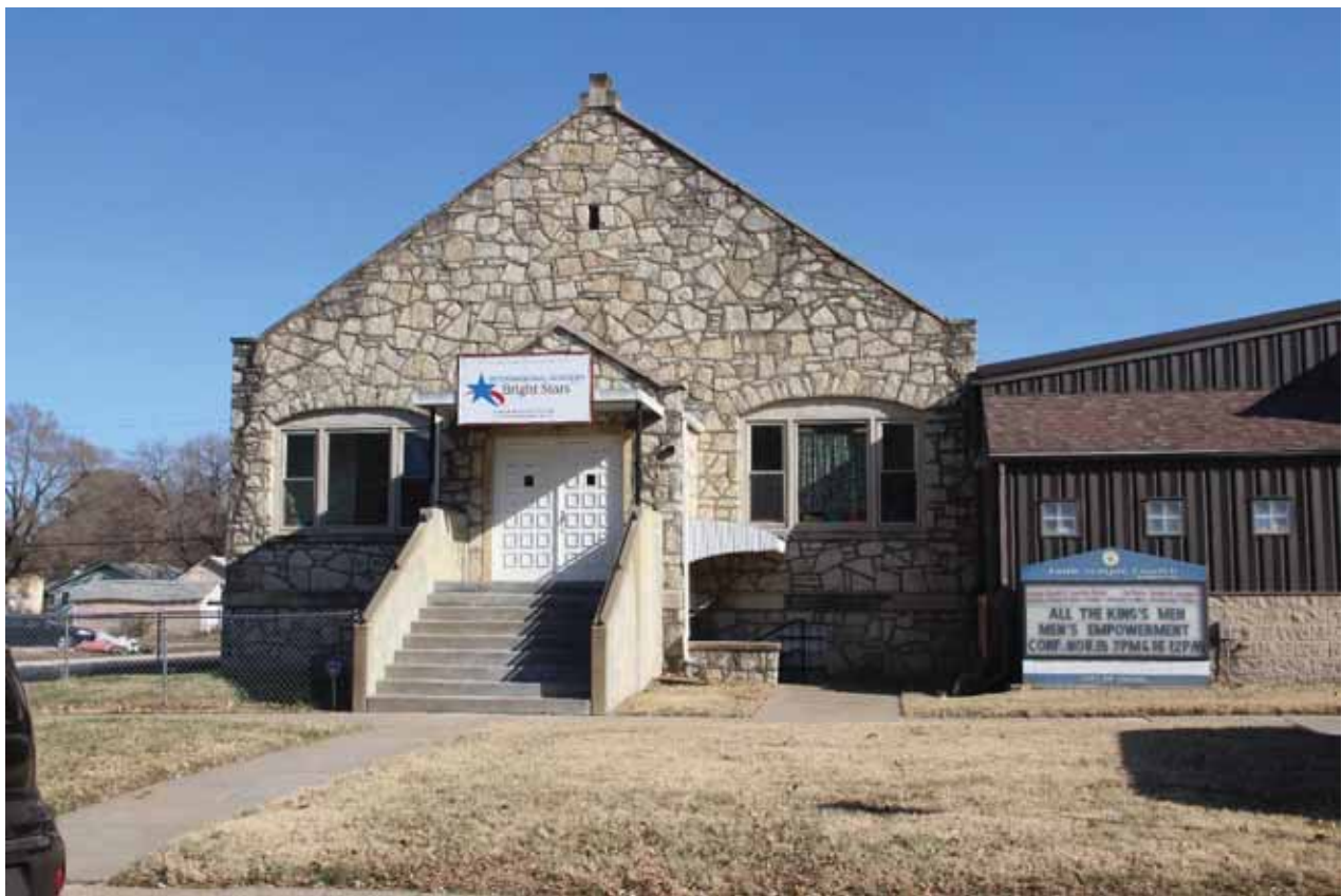
Figure 30. 1162 SW Lincoln Street is an Ozark Giraffe stone church constructed in 1951 (Photo: Keenoy, 14 November 2019).
