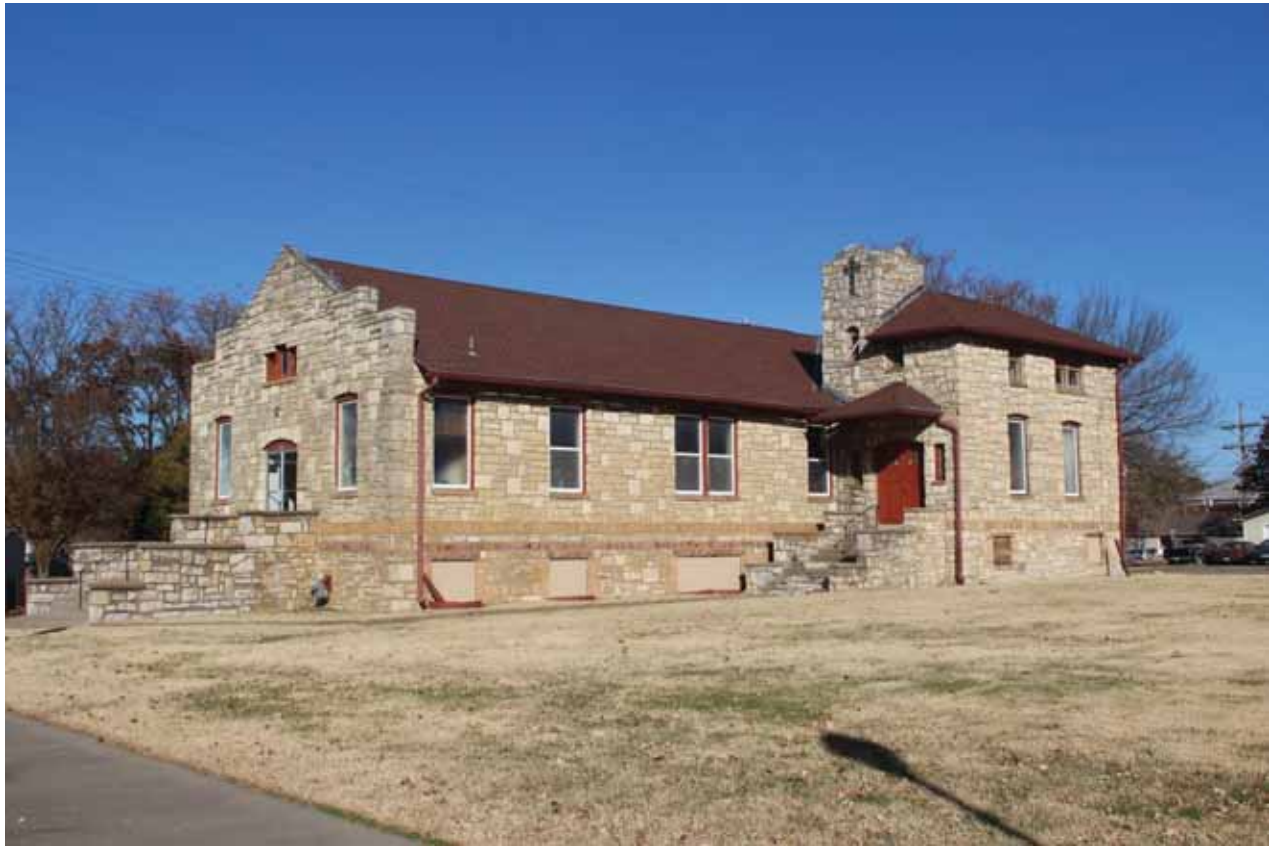
Figure 35. Lane Chapel at 1200 SW Lane Street is an excellent example of a Mission style church that supported the African-American residents of Tennessee Town.
