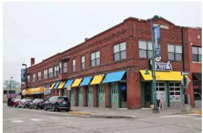
The J.L. John’s Building at the corner of 12 th and Moro Streets is a good example of a traditional historic commercial building. The building retains its historic shaped parapet and brick corbelling on the parapet as well as paired windows on the upper facades. The 1918 building was constructed with multiple storefronts at street level and apartments on the upper floor. The storefronts have been modified and replaced on numerous occasions, the latest introducing operable vertical bi-fold and horizontal-light operable windows which are not compatible with the building’s historic character. However, the storefronts maintain historic proportions and fill the original openings. With the intact upper facade, the building retains sufficient integrity to convey its historic commercial design and function. Similar windows on a one-story building may diminish the historic character to a degree that the building is not eligible for historic listing.
