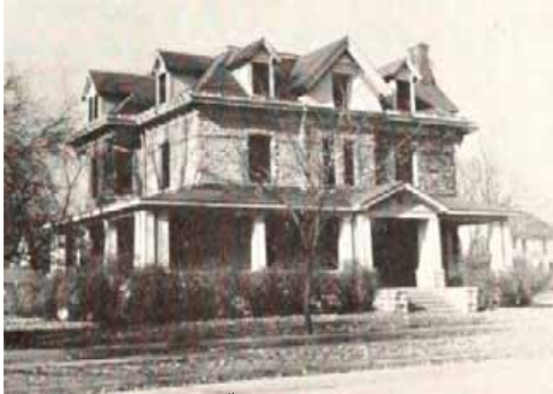
Hessin House at 519 N. 11 th Street built in 1886 (1936 Royal Purple).
