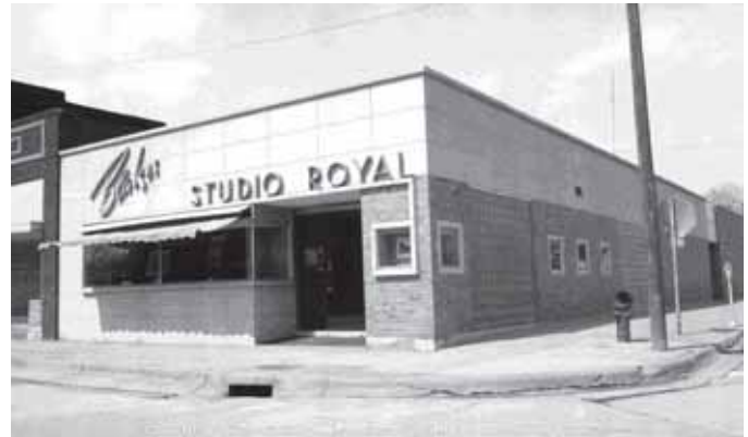
Blaker Studio Royal at 1200 Moro St. was built in 1946. This concrete block building features an asymmetrical facade of smooth ashlar stone and light-colored brick. The design had glass block bays on the east street facade, likely to provide indirect lighting in the photo studio. The building retained its historic appearance in this 1979 photo but has since been remodeled, losing much of its mid-century character (1979 Historic Survey, RCHM).
