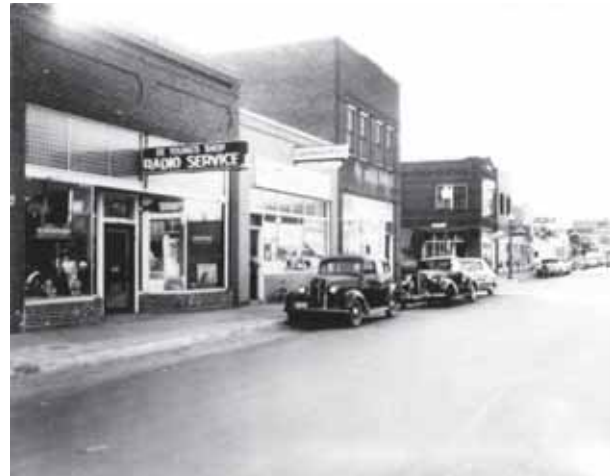
DeYoung's Radio Service moved to 1127 Moro St. from the Wareham Building and Henry Miller built the existing building at 1129 Moro St. in 1947 to house a launderette (Riley County Historical Museum).
