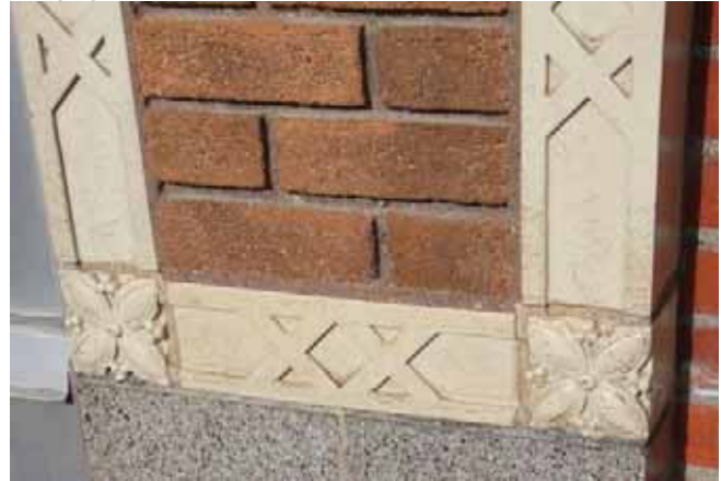
Terracotta detailing on Forrester Building at 1218 Moro Street.
