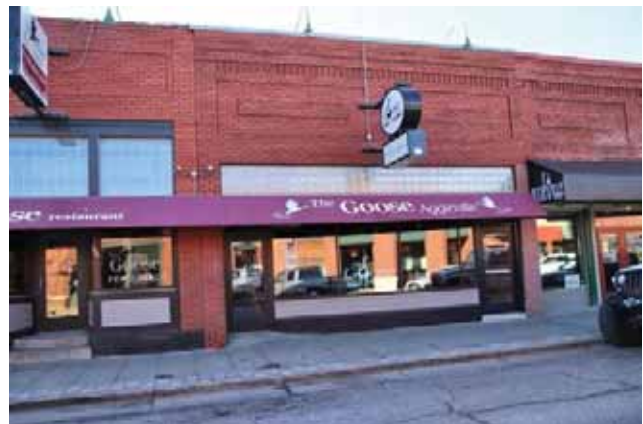
These three one-story brick buildings located at 1123- 1127 Moro St. are among the district's earliest existing commercial buildings built in 1912. They are classic representatives of the Commercial Style with brick facades featuring corbelling on the upper facade as the only ornament.
