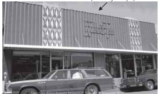
Aluminum slipcover extant in 1979 Historic Survey photo ( RCHM).
