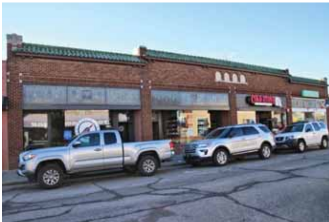
Built in 1926, the Wareham Building in the 1200 block of Moro St. exhibits the classic form of a Commercial Style building with brick piers framing multiple storefront bays. The use of green clay tile at the parapet illustrates Spanish/Mission Revival style influences.
