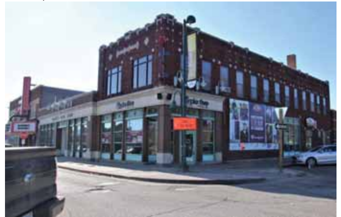
Current view looking SW on N. Manhattan Ave. with former Varney's buildings and theater. Prior to closing in 2016, Varneys had expanded into three buildings on the south. The existing storefronts and first-floor facades on the northern three buildings date to a 1989 remodel that compromised the historic integrity of the buildings. The building(s) between the theater and the bookstore were originally two separate buildings occupied by College Drug/Miller Pharmacy and Duckwall's/Bottger's IGA. Other than replacement of the stone panel on the parapet, the remodeling of the theater for Varney's bookstore in 2013 retained the upper facade and theater marquee – historic features that distinguish the original theater building. Even though these buildings have lost some historic integrity, the bookstore and theater would be contributors to a historic district and are long-time businesses that hold an important place in Aggieville's history.
