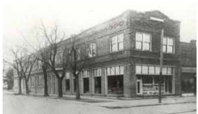
J.L. John's Confectionery built at 1201 Moro St. in 1918 and L.C. Shafer's Grocery at 1203 Moro St. was built in 1915 as a one-story building (R) and expanded to two-story in 1923 (Dan Walter, Aggieville Archives).
