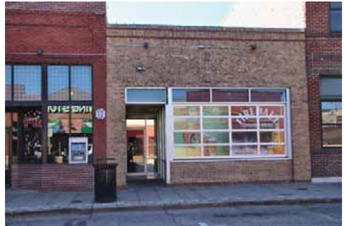
Miller Launderette built in 1938 at 1129 Moro St. reflects the Minimal Commercial style with its blond brick facade, minimal ornamentation, and punched storefront opening.
