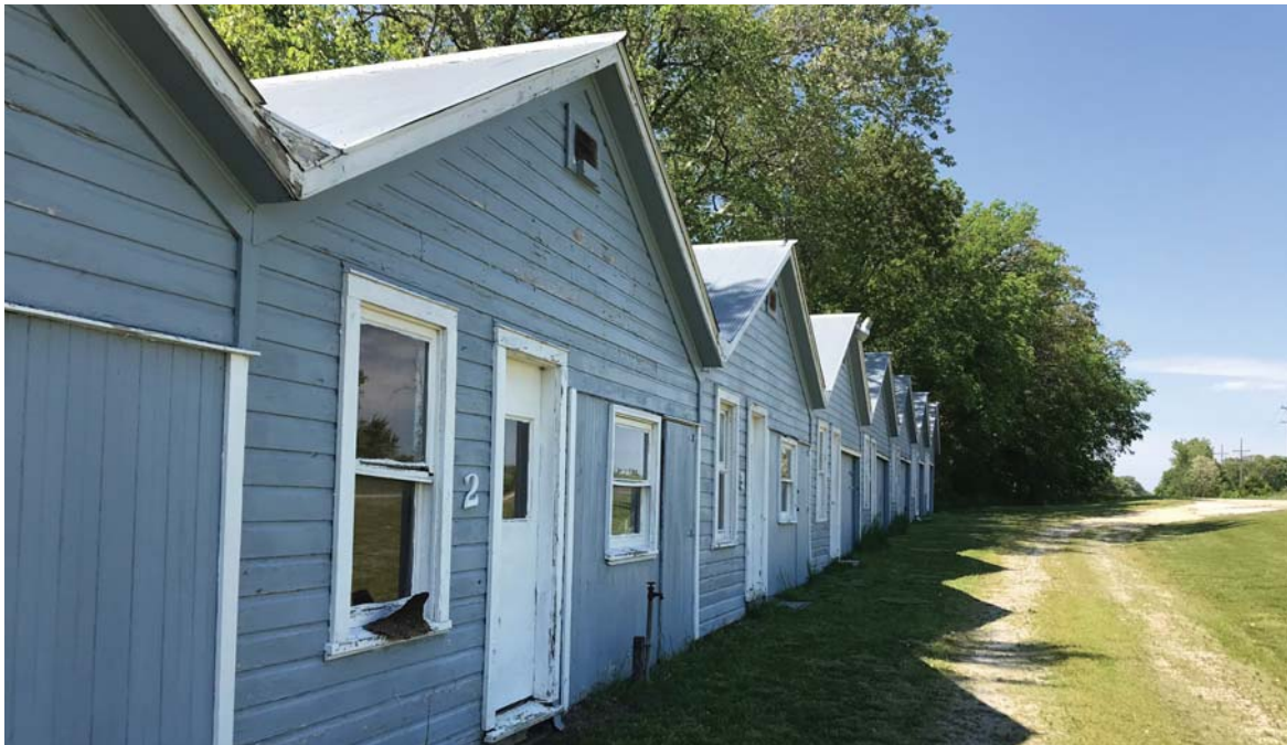
Dyer Cabins was built in the 1930s as a Motor Court/Motel. Properties like this that back up against a creek or river are not as common in Kansas as they are in Missouri. This one is relatively unchanged from its original construction and appears to be eligible for listing. Photo by Christy Davis, 2019.
