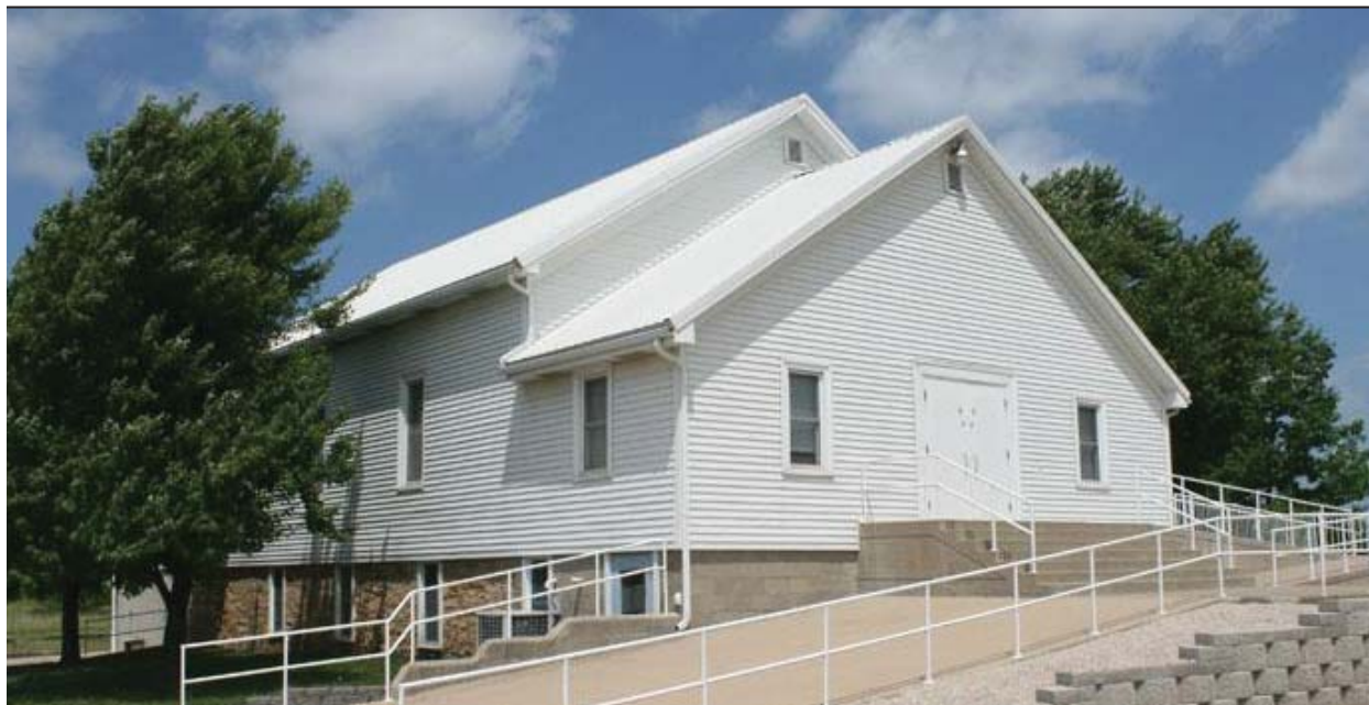
The Old German Baptist Brethren Church is still active in Willow Springs today. Their meeting place, constructed in the late nineteenth century, has been expanded over the years. KHRI. Photo by Susan Ford.
