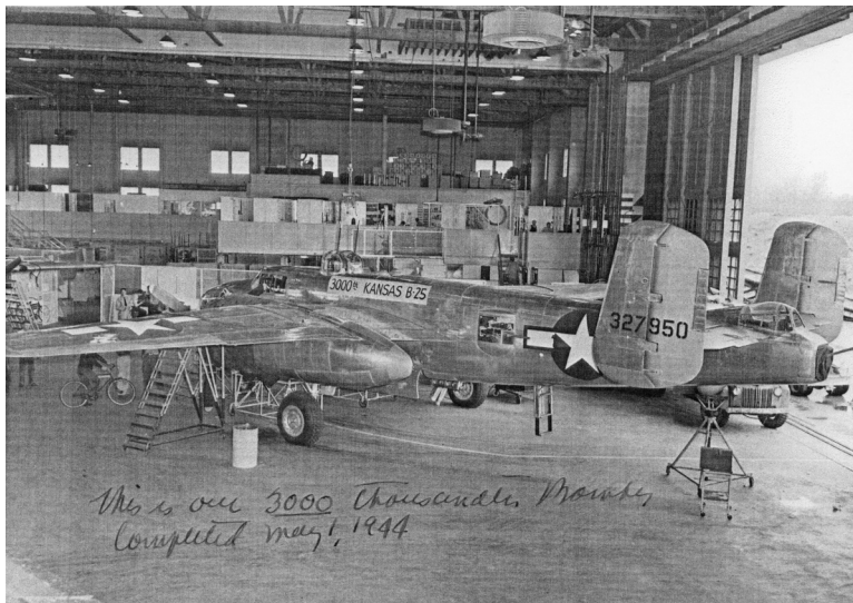
In December 1943 the Kansas facility began production on the B-25J; number three thousand is shown here. Among other changes, the NAA did away with the retractable bottom turret, moved the top turret forward near the pilot's compartment, and added armor protection for several crew positions. Courtesy of the Wyandotte County Museum.
