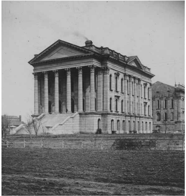
This 1880 photograph shows the east and west wings of the Capitol in Topeka, Kansas. Ten years earlier, two different views of democratic governance clashed in the unfinished structure's courtroom. The fundamental question underlining Craft v. Board of County Commissioners of Jackson County, Kansas , was that of an individual's place in a community and his or her ability to direct its course.
