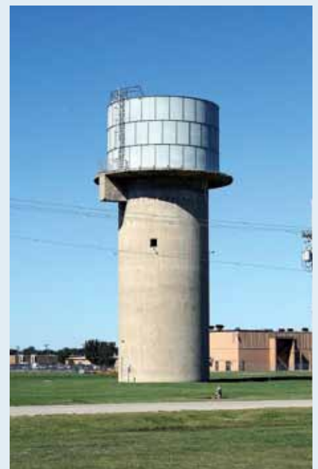
1940s Coffeyville AAF Water Tower
