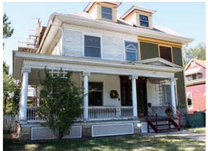
The P.N. Randal House is currently undergoing renovation.
