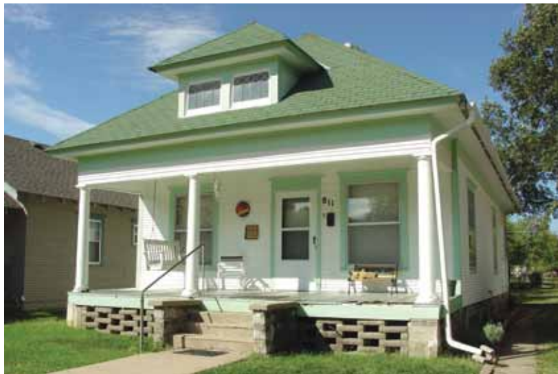
One-story cottages can be found throughout the south central neighborhood.
