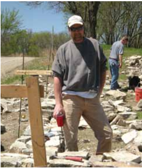
Left to right, Rocky Slaymaker led the workshop near Alma; string lines serve to guide builders to create a fence that is battered—wider at the bottom than the top, workshop participants continuing rock wall restoration from 2010.
