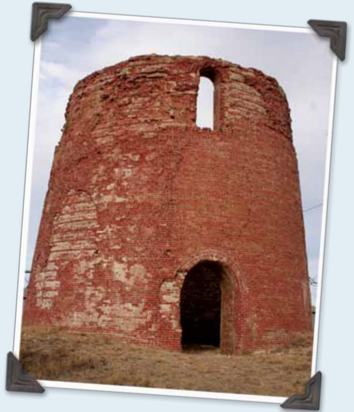
1887 Coolidge Water Tower
