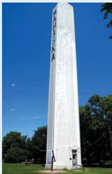
1930s Mahaska Water Tower
