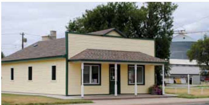
There are still a handful of false-front buildings in Gray County. This one in Copeland likely dates to the time of the town's founding in 1912. Photo courtesy Christy Davis.
