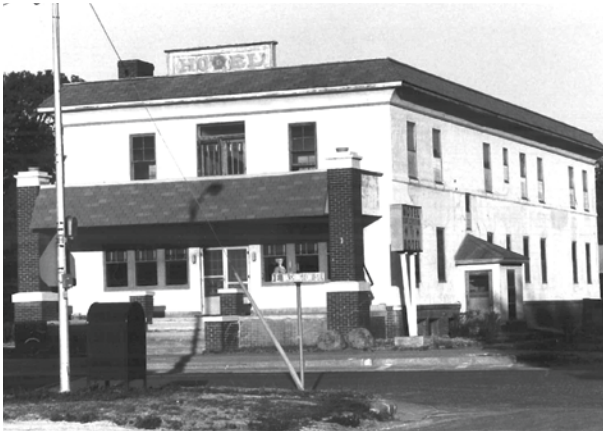
Sunflower Inn, Osborne Built 1924; demolished September 2014
