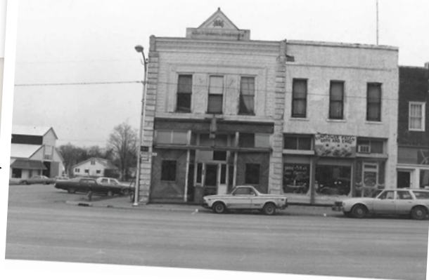
731 (Left) - 729 (right) Wisconsin Street, Cawker City Built 1889; listed 1986; demolished spring 2014
