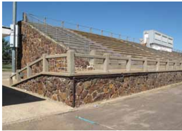
Martin Stadium, Salina Built 1940; demolished April 2014
