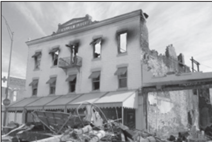
Plans call for stabilizing the Miller Block, the oldest building on Main Street.
