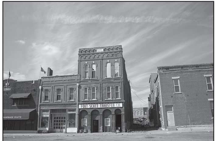
The Fort Scott Transfer Building, damaged in the fire, was constructed in the 1870s to serve as the Odd Fellows Hall.
