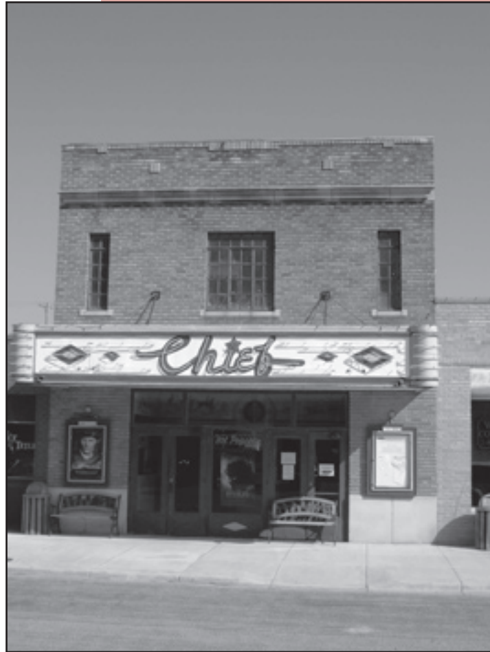
Built in Coldwater in 1928, the Chief Theater typifies the two-part commercial block movie theater.
