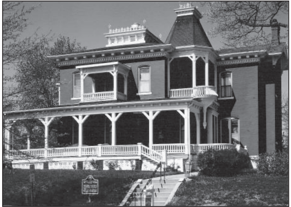
A $28,800 grant to the Leavenworth County Historical Society will fund roof repairs to the Carroll House, a living museum and home the the LCHS.
