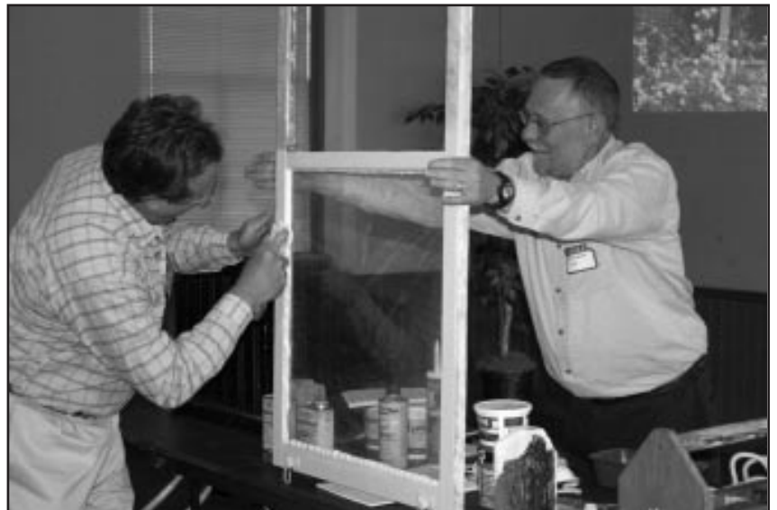
Lawrence contractors Dennis Brown and Mike Goans demonstrate how to properly glaze a wood window.
