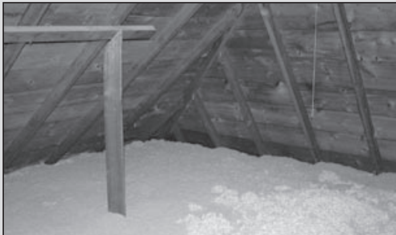
Cellulose insulation, made from recycled materials, is a good choice for insulating unoccupied attic space.
