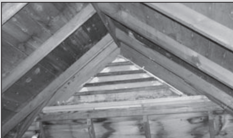
Louvers and vents help keep your attic properly ventilated so moisture does not cause deterioration.
