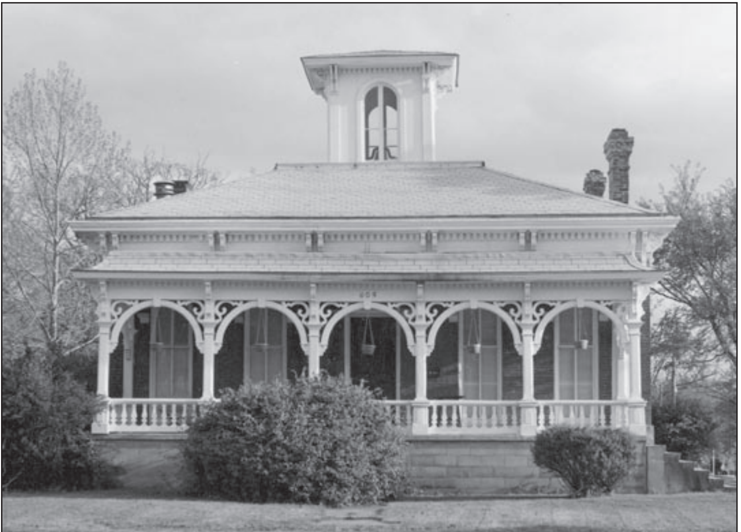
The Niles House is an excellent example of Italianate architecture.
