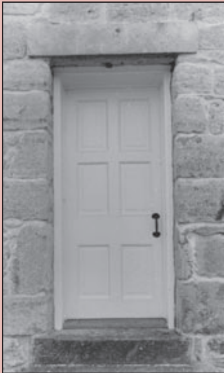
An exterior door boasts a fresh coat of paint.
