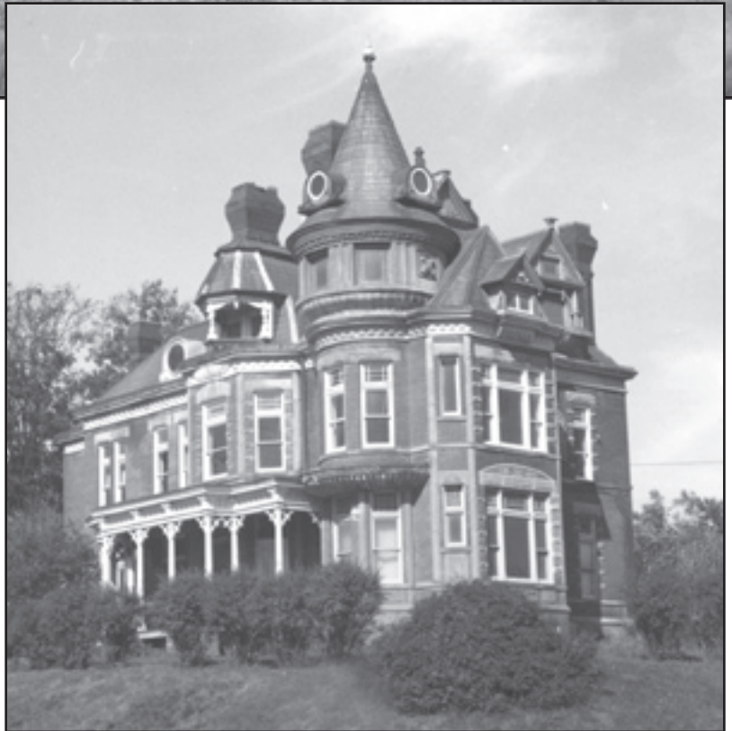
Atchison's McInteer Villa (c. 1889-1890) is a rare and elaborate interpretation of a masonry Queen Anne. Most Queen Anne examples were built of wood.
