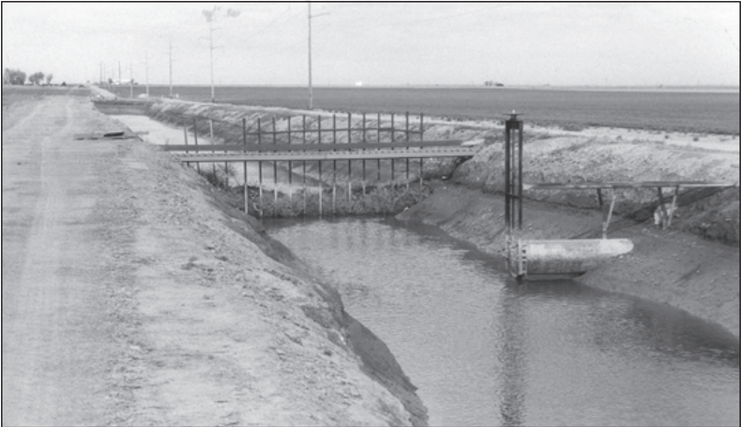
Current west view of the Great Eastern Ditch and operating machinery at Big Lowe and Rodkey Roads. Photo by Susan Ford.
