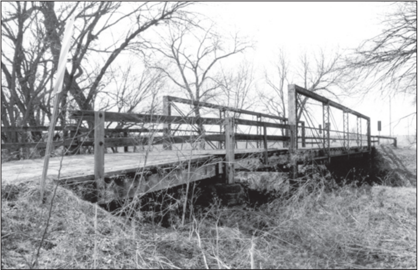
The Hobbs Creek Truss Leg Bedstead Bridge near Gypsum in Saline County was constructed by the Missouri Valley Bridge Company in 1907.
