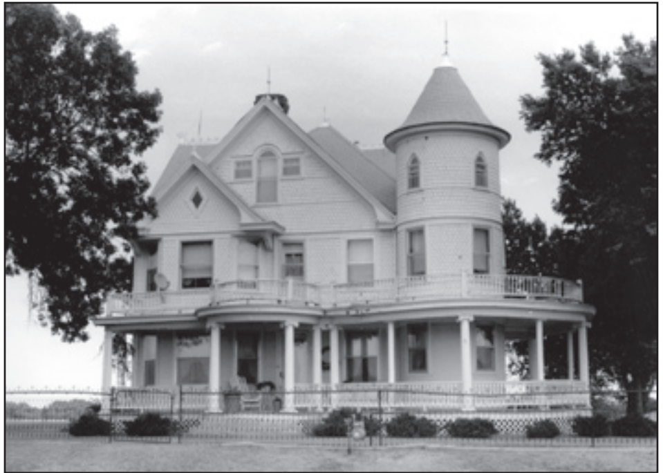
Free Classic Queen Anne houses use classical columns rather than delicate, turned posts with spindle work detailing as porch supports. Palladian windows, cornice-line dentils, and other classical details are frequent. The photo shows the O. W. Francis House near Burr Oak.
