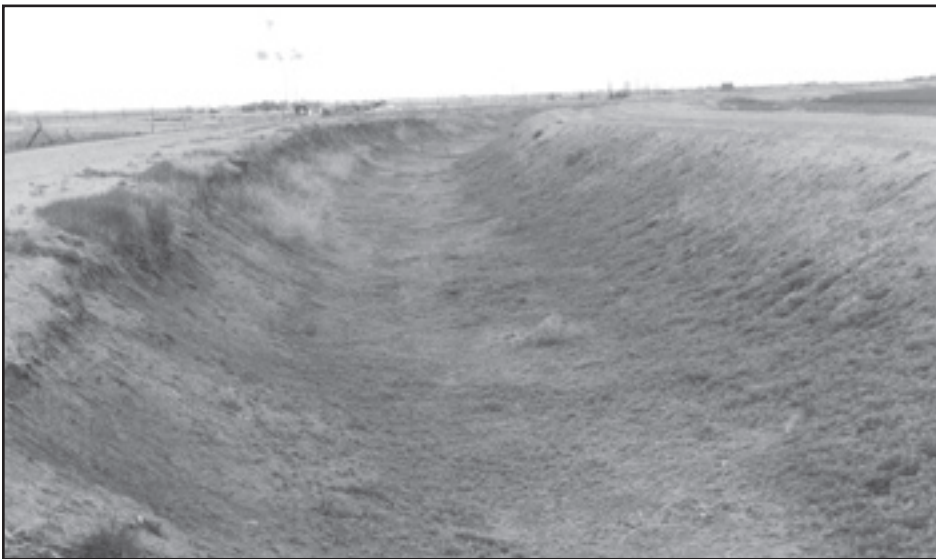
Current west view of the Farmers' Ditch west of US-50 on VFW Road. Photo by Susan Ford.
