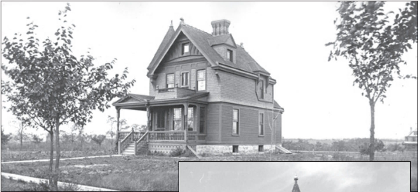
A typical late-nineteenth-century Queen Anne style house featured various kinds of machine-made shingles, wooden ornamentation for the porches, and an elaborate chimney. This ca. 1890s photograph shows the Marbury House at 429 Greenwood, part of what is now the Potwin Place Historic District in Topeka. Photo from the Kansas State Historical Society collections.
