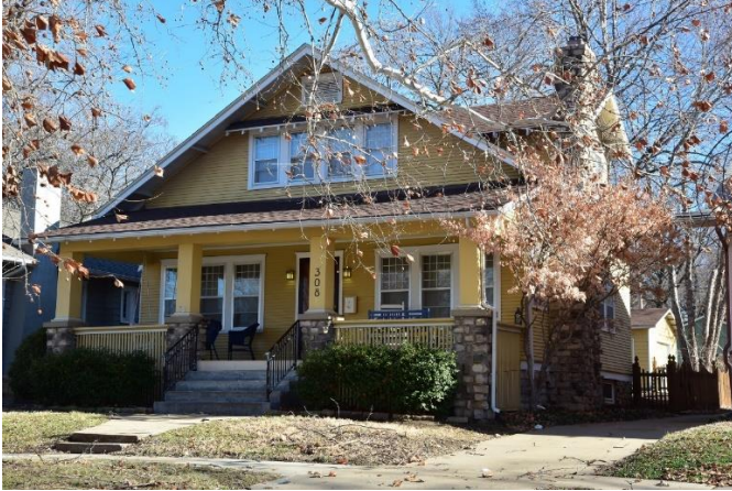
Figure 10: 308 SW Elmwood Avenue, Topeka, Kansas. Source: Brad Finch, 2019
