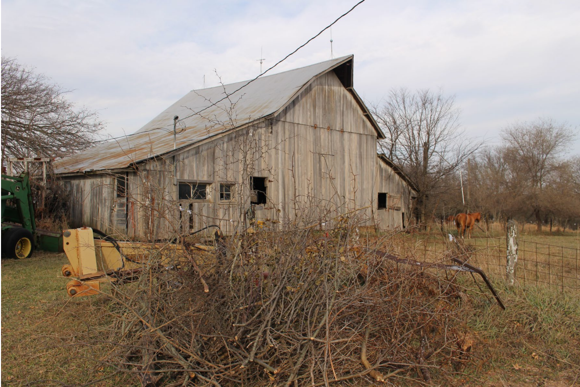
Photo 1: Exterior of the Barn, 2019
