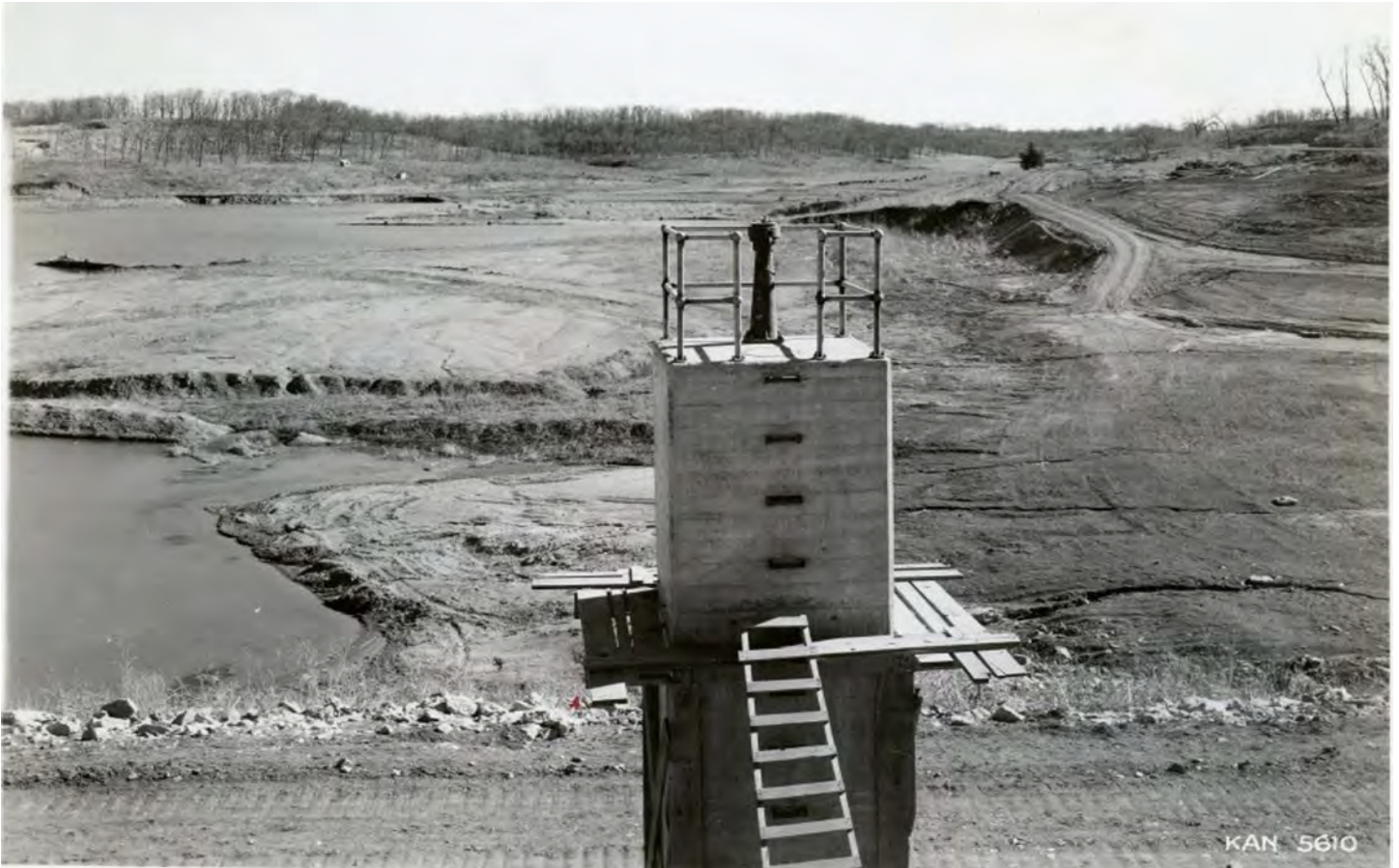
Figure 10: Historic Photo of Lone Star Lake Dam & Lake under Construction, looking south at the control outlet tower. Unknown Date. Image provided by the Watkins Museum of History
