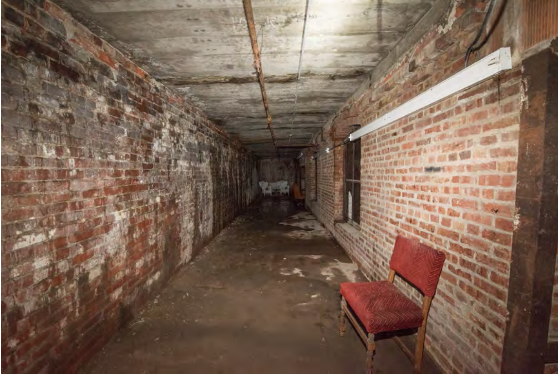
Photo 9: Basement, looking north from south end of west storage area
