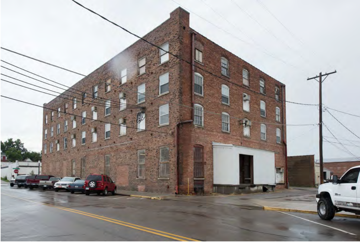
Photo 3: Looking northeast at west and south elevations
