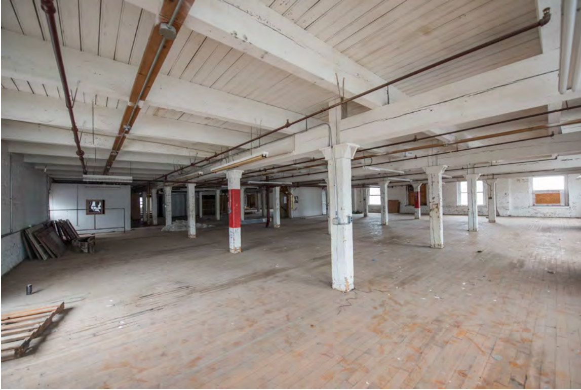
Photo 5: Second floor, looking southwest from northeast corner of floor
