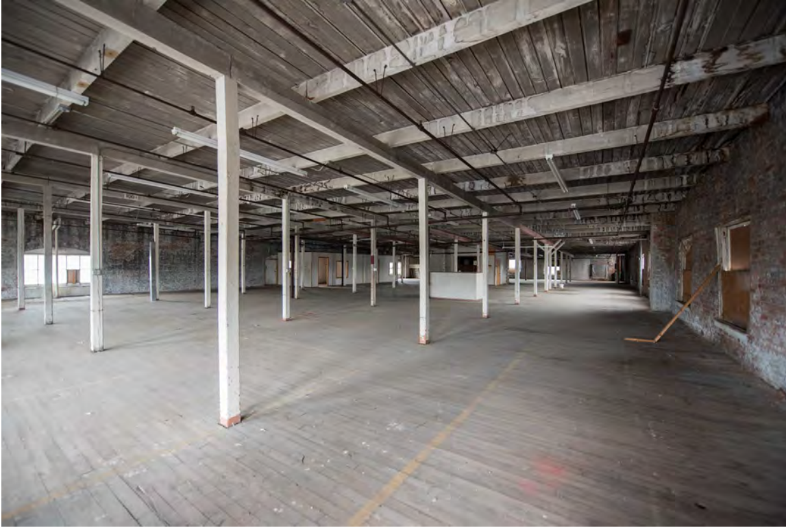
Photo 7: Fourth floor, looking southeast from northwest corner of floor
