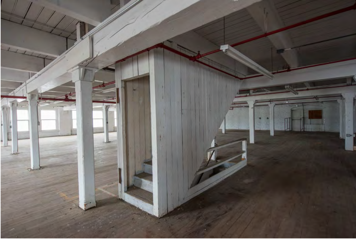
Photo 11: Third floor, stair core, looking northeast
