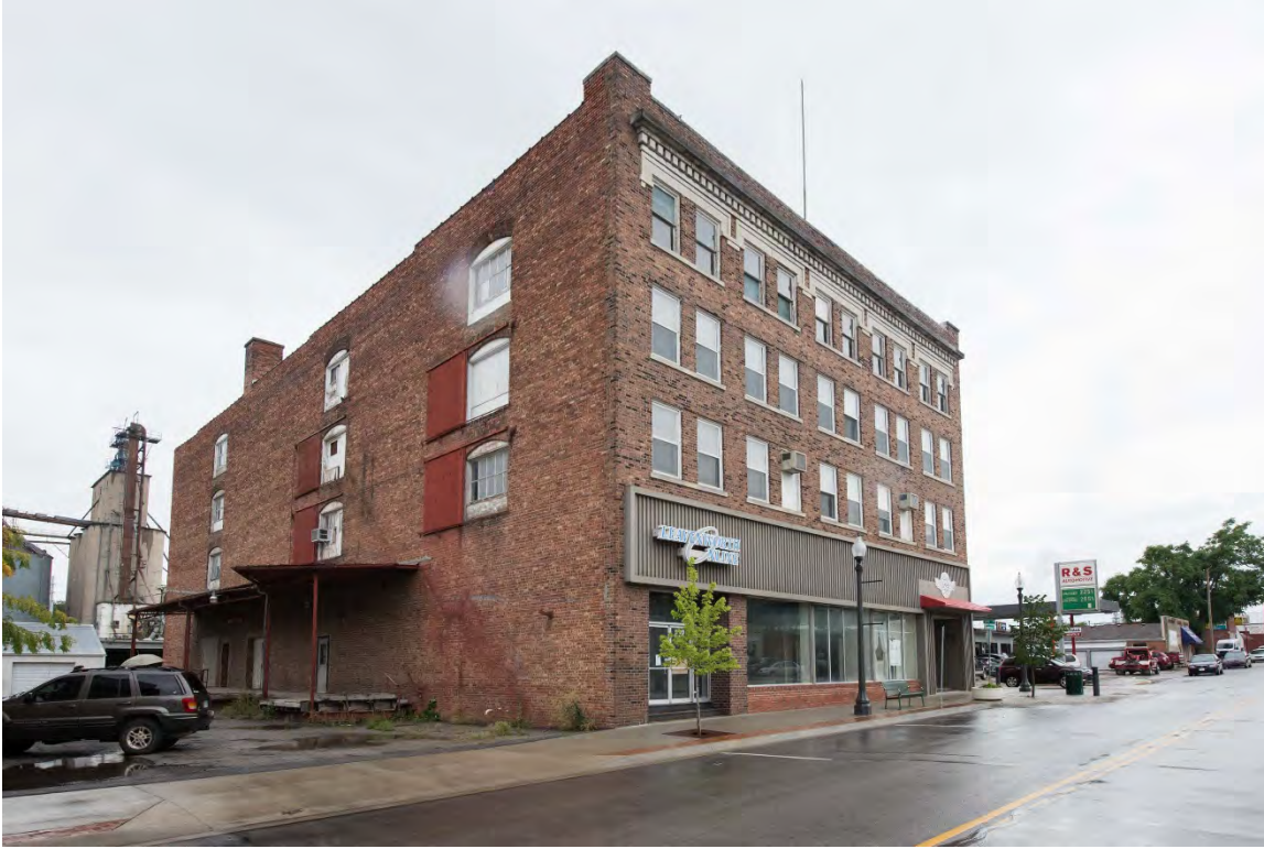
Photo 1: Looking southwest at east and north elevations
