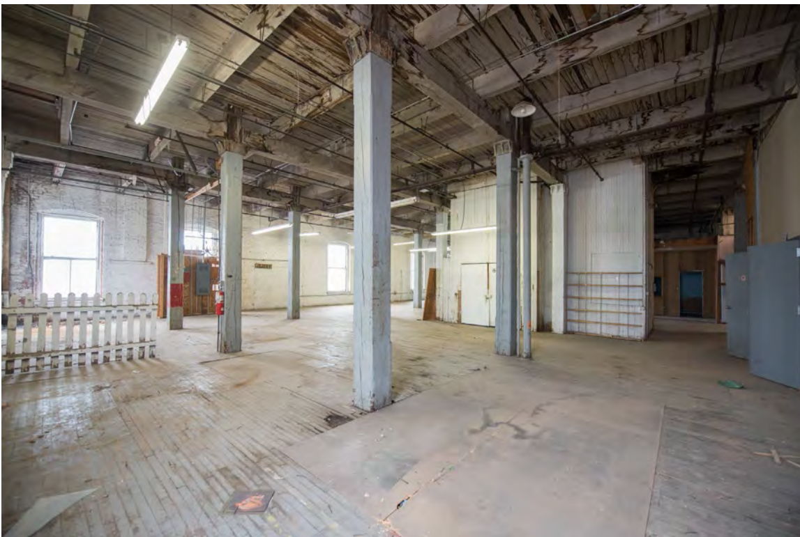
Photo 4: First floor, warehouse area at rear of building, looking northwest
