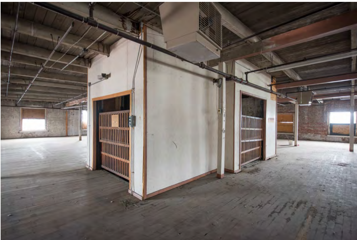
Photo 10: Fourth floor, elevator core, looking southwest
