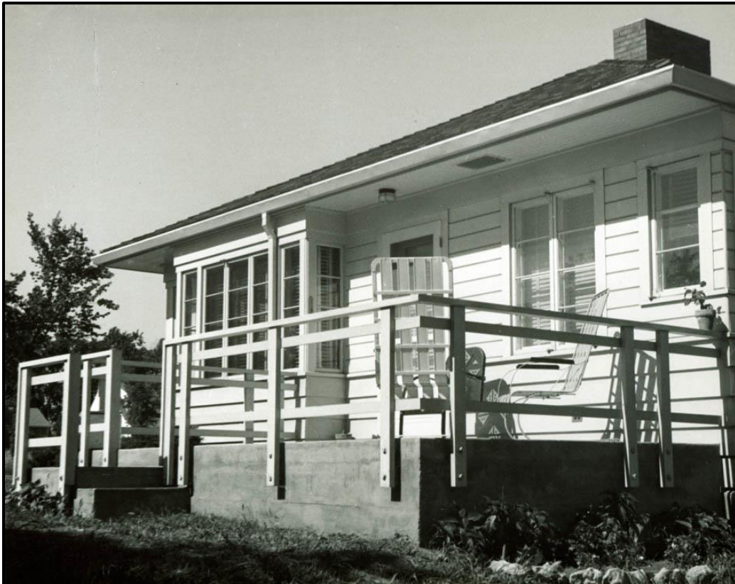
East Façade from Northeast
