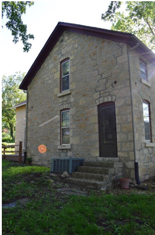
Figure 4. West elevation viewed to the east, original portion of the residence
