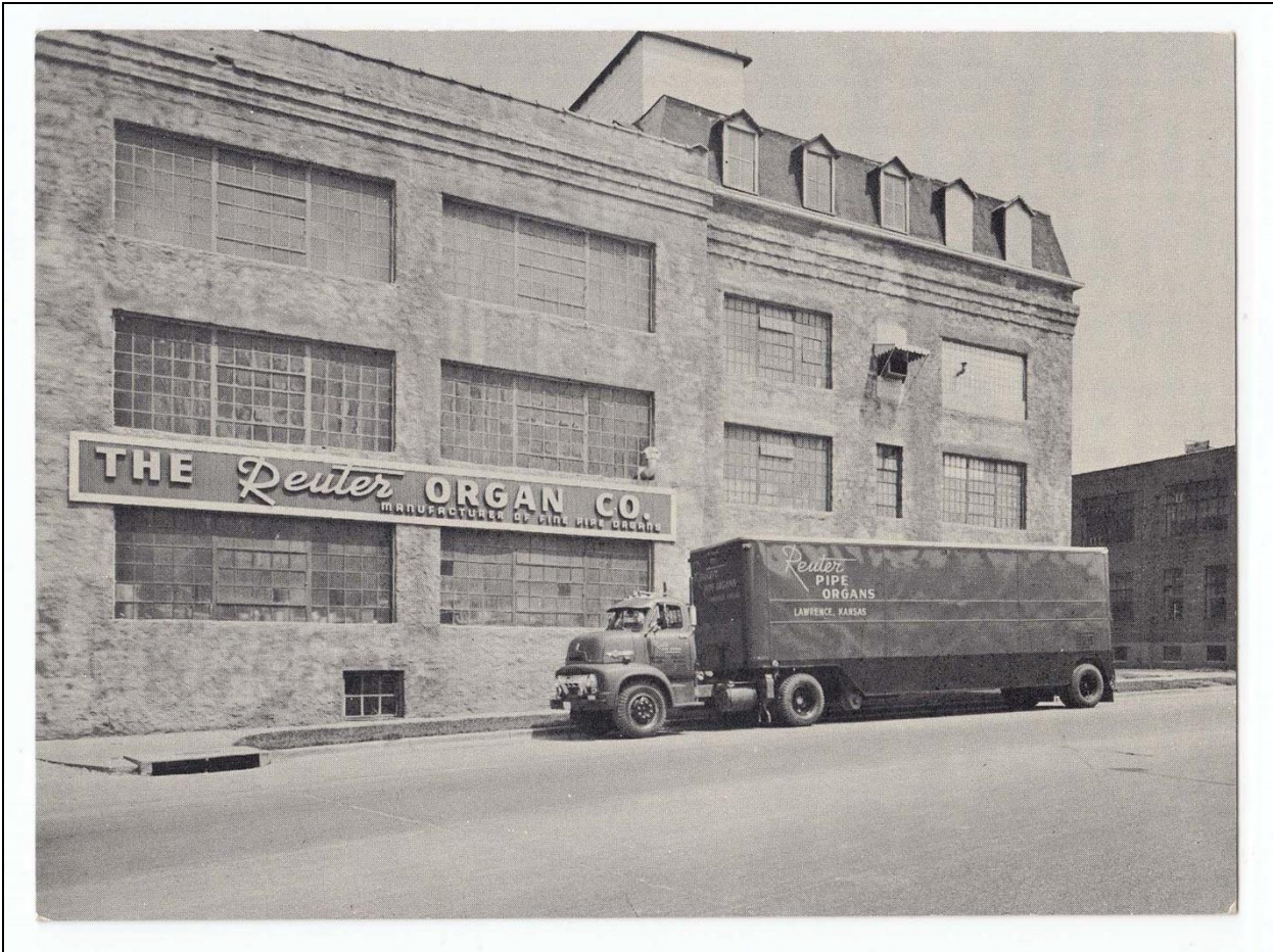
Figure 6. Circa 1956, showing glass block window unit.
