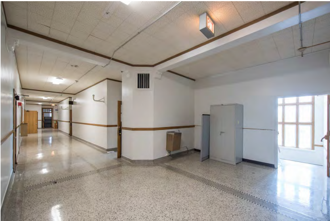
Photo 10: Second floor corridor (1926 building), facing northeast
