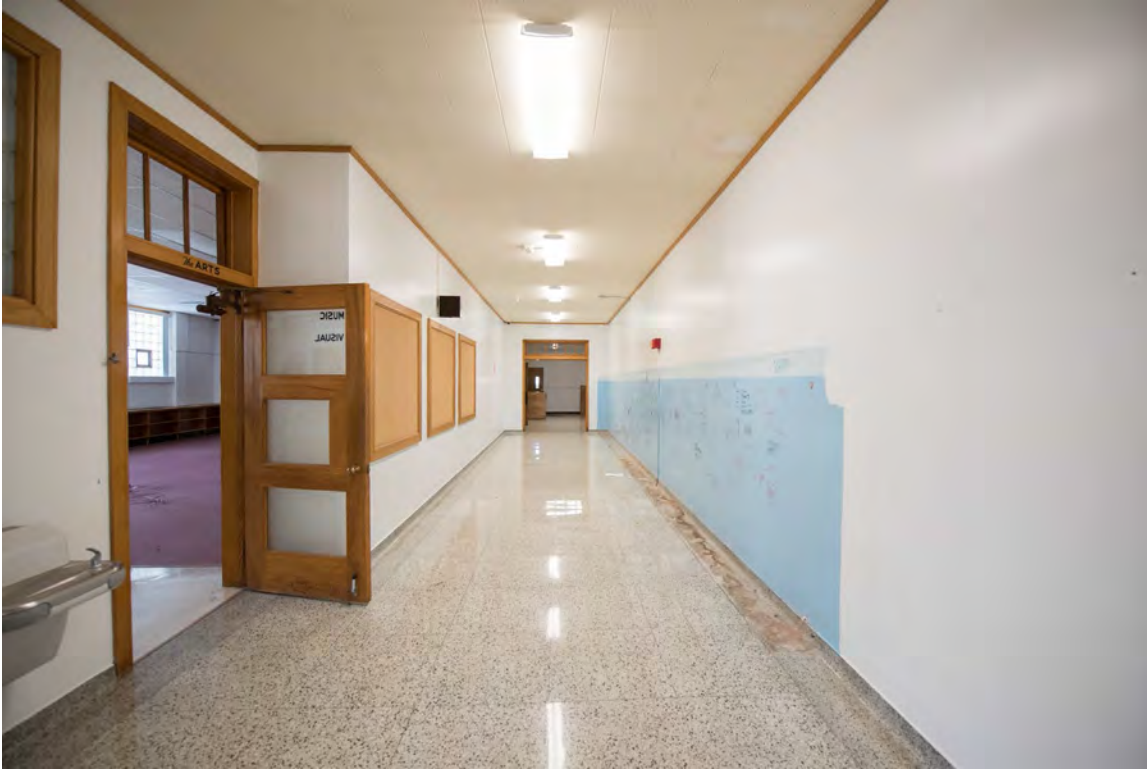
Photo 11: Second floor corridor (1951 addition), facing east
