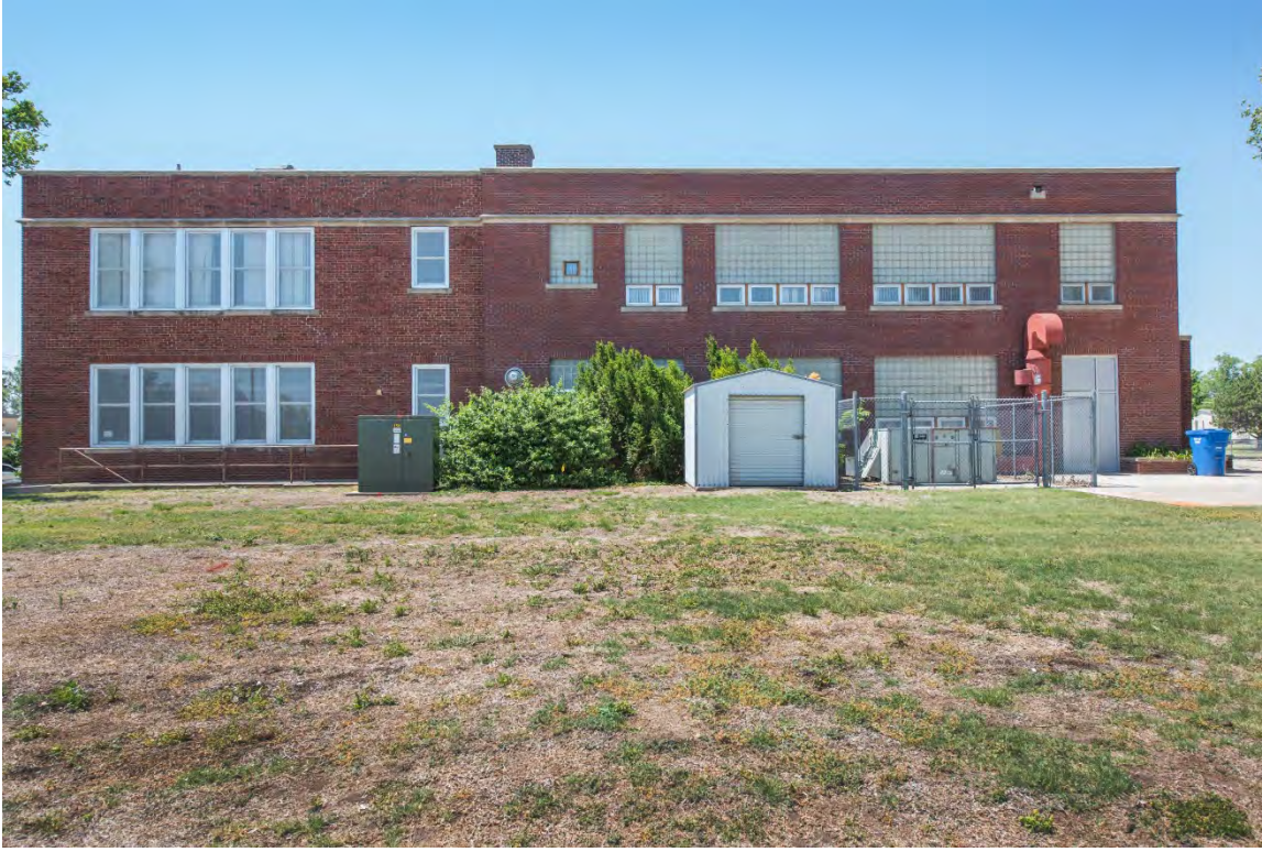
Photo 5: North elevation, facing south
