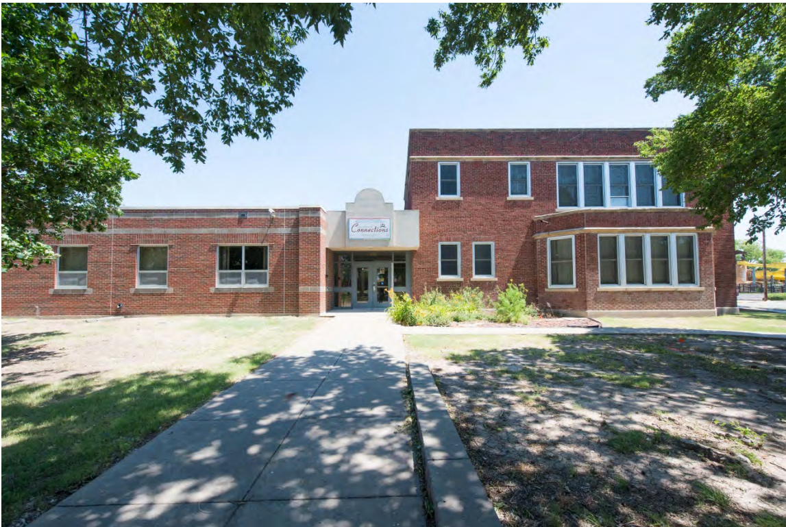
Photo 8: South elevation, facing north
