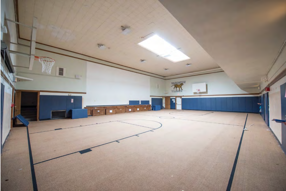
Photo 15: 1931 Gymnasium with view of covered proscenium, facing northwest
