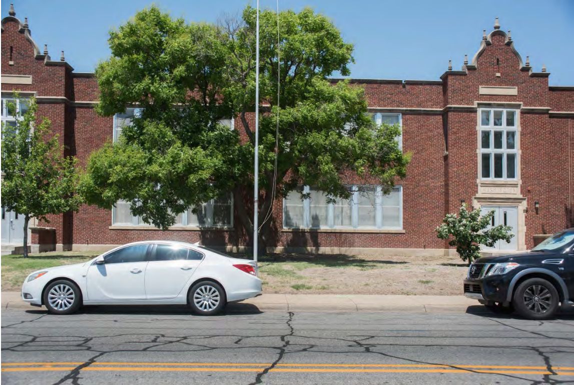
Photo 1: Front (east) elevation, northern entry, facing west
