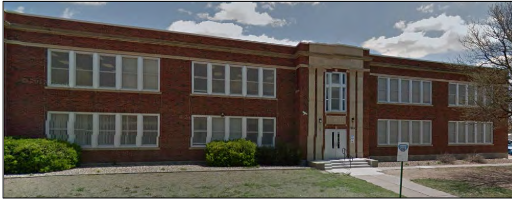
Figure 8: 1925 portion of Lincoln Grade School. Source: Google Streetview.
