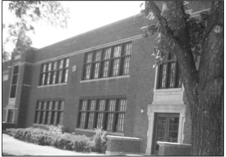
Figure 02: 1970 Survey photograph showing historic muntin configuration.
