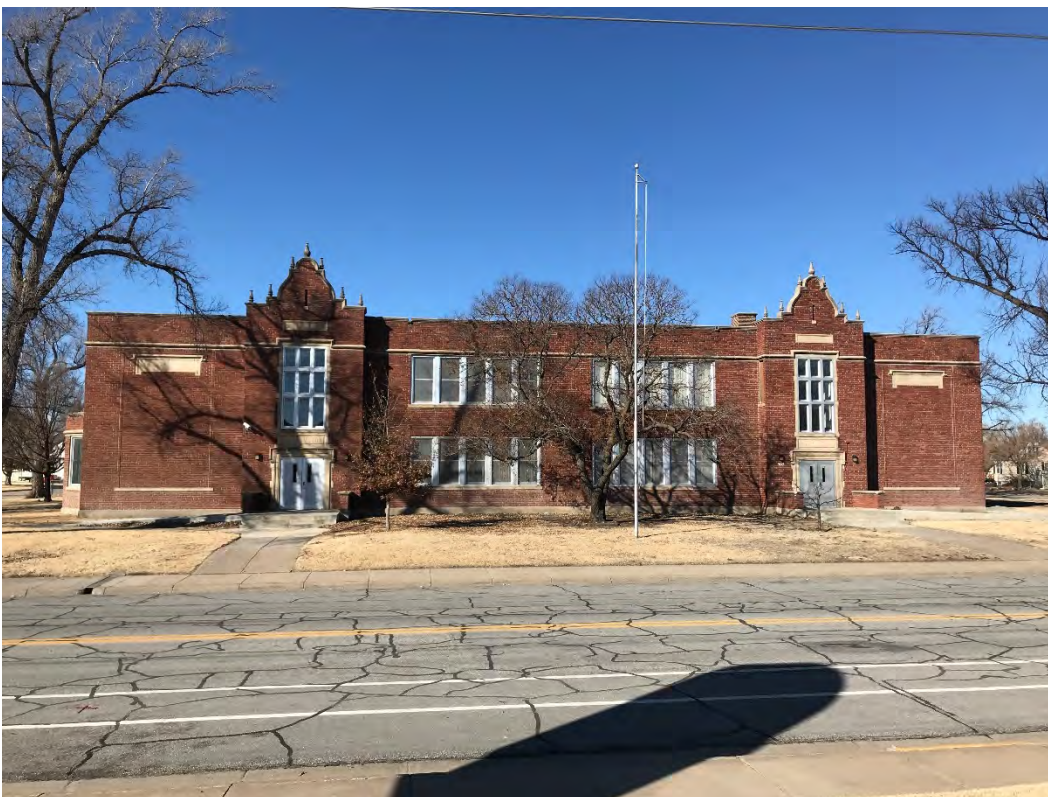
Photo 18: Full front (east) elevation, facing west, photo from JRG Architects, Spring 2020
