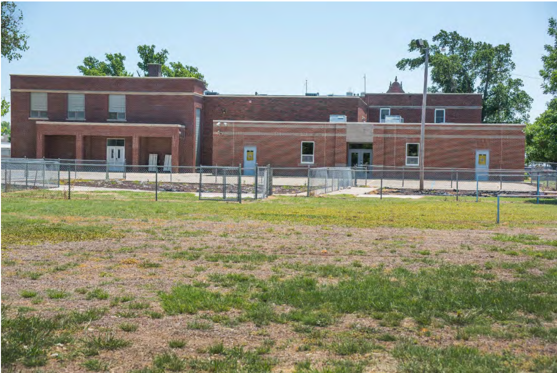
Photo 6: West elevation, facing east
