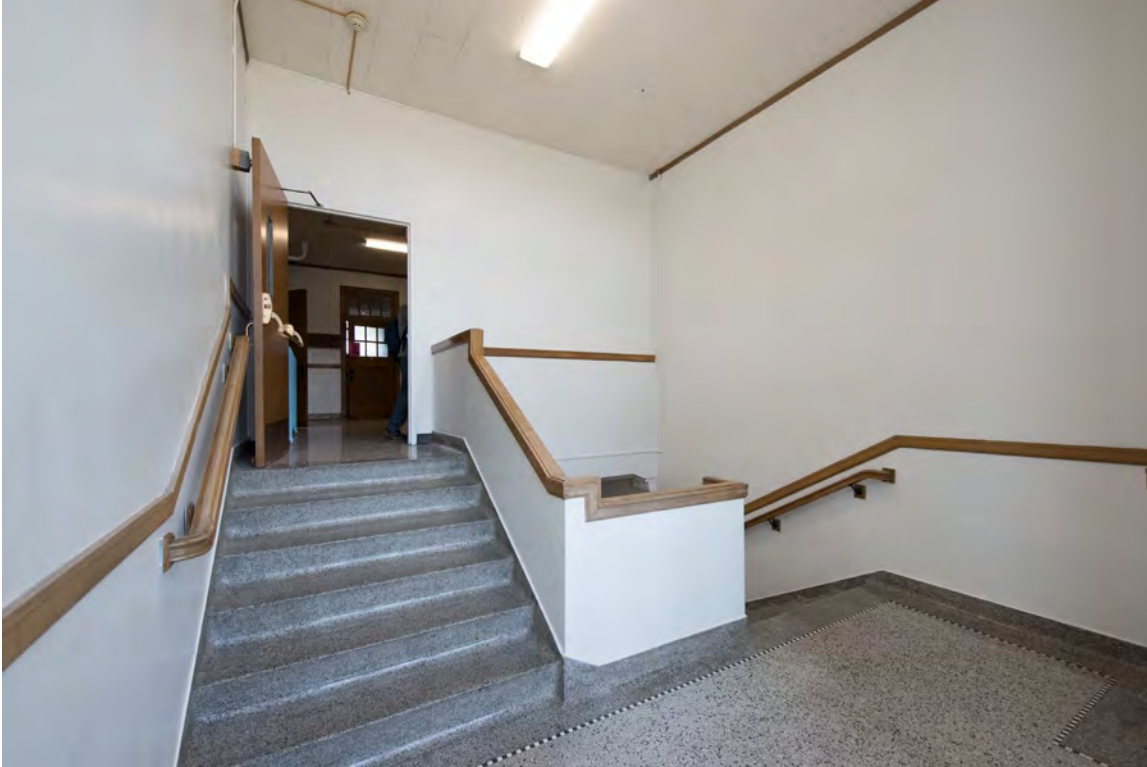
Photo 9: 1926 Building, south stair, landing between first and second floors, facing northwest
