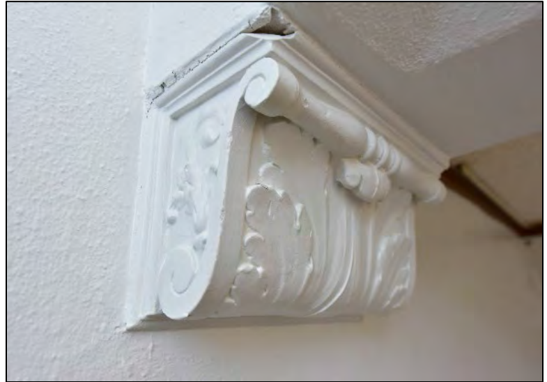
Figure 03: Typical plaster scroll bracket. Photo: Brad Finch, 2020.
