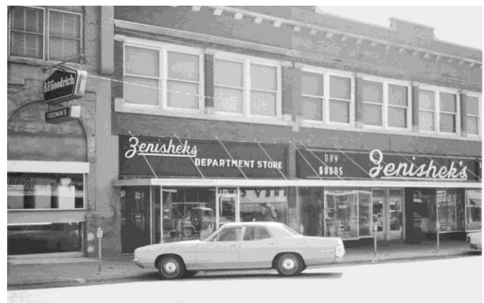
Figure 23—Crebo Building reconstructed after 1937 fire (#63-62-61)
