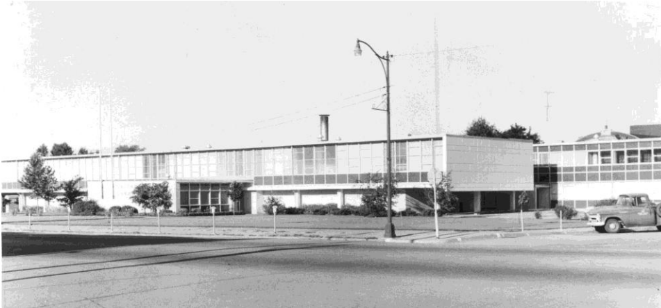
Figure 5 – ‘New’ courthouse dedicated 1957 on site of old courthouse in 300 block of N. Main (Building #1)
