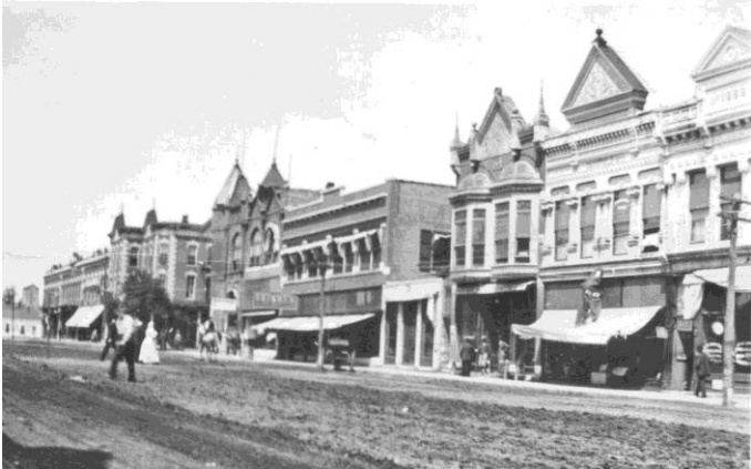
Figure 20—East side of the 200 block N. Main (Bldgs #57-65)
