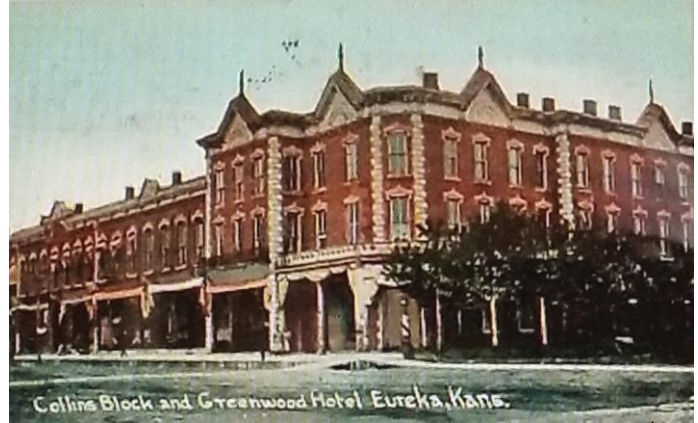
Figure 21—Greenwood Hotel (Building #65) at NE corner of 3 rd & Main
