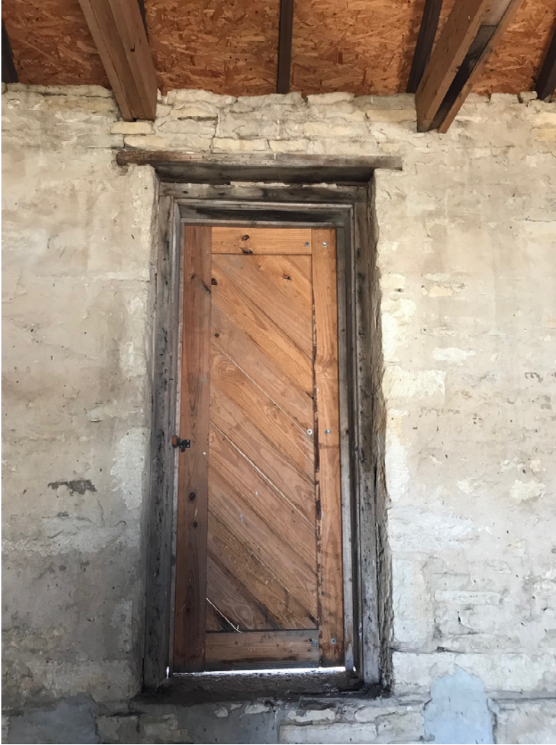
Figure 10: Interior of Limestone Outbuilding showing possible former floor framing.
