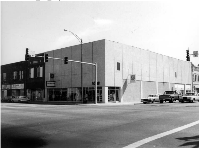
Figure 11 - 1991 View after Otasco vacated building. They installed the aggregate panels over the brick facade when they opened in the building in 1965. (Photo by Wichita Metro-Area Planning Department downloaded online at https://khri.kansasgis.org/ )
