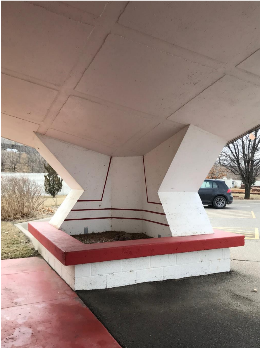
Photo: One of the two large column planters at which the roof shell terminates.
