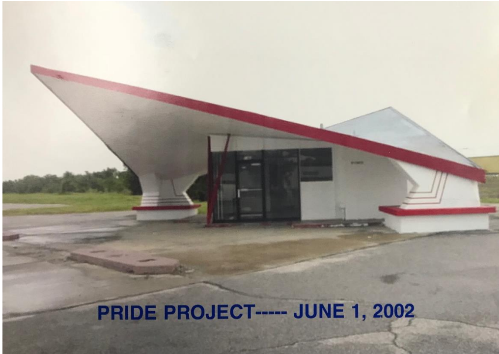
Figure 5: After the Pride Project in 2002. A first reconstruction was built in 1999 with a wood-framed bulkhead above the storefront. Volunteers painted the building as part of the Pride Project. Photo courtesy of Rosemarie Corby.
