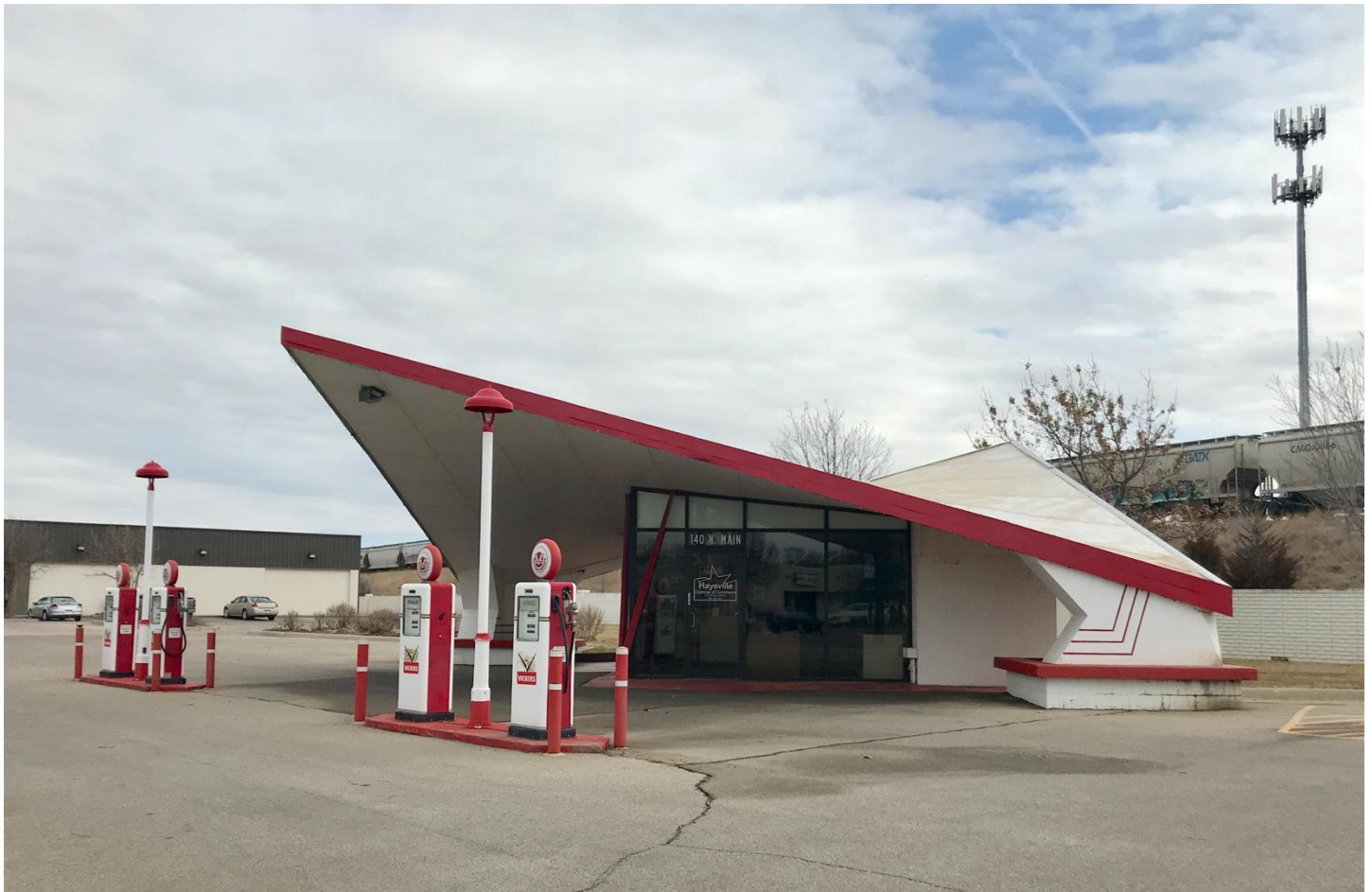
Photo: The two axes of the building can be observed. The batwings open to the east and west.
