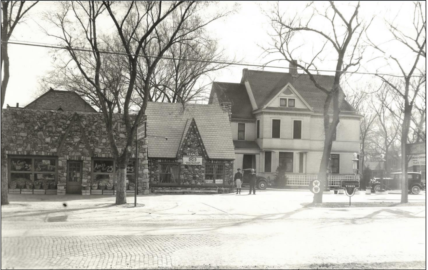
Figure 4: Taken from north of the property on 6th Avenue, looking south, ca. 1935.
