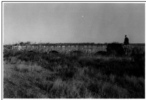
North Fork Walnut Creek Tributary Bridge, Beeler vicinity (ca. 1941). Only known quadruple arch in county.
