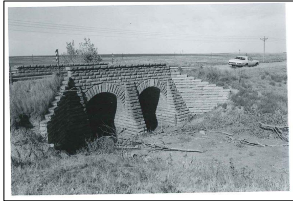
Pawnee River Tributary Bridge, Bazine vicinity (ca. 1928). NR-listed, 1985.
