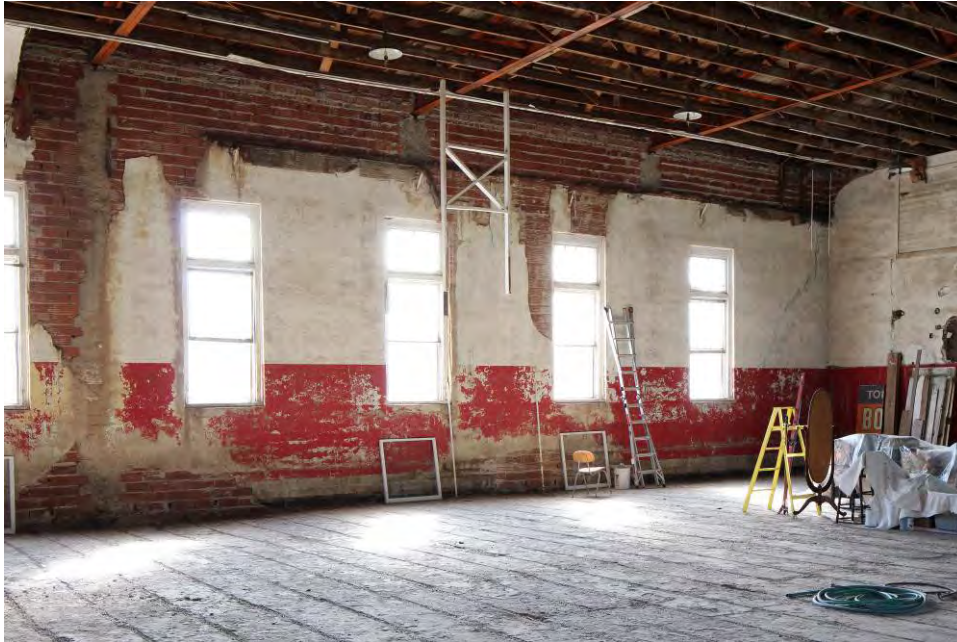
Photo 12: Looking SE, east wall
