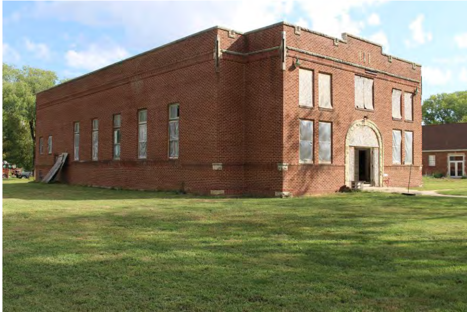
Photo 5: South and west elevations
