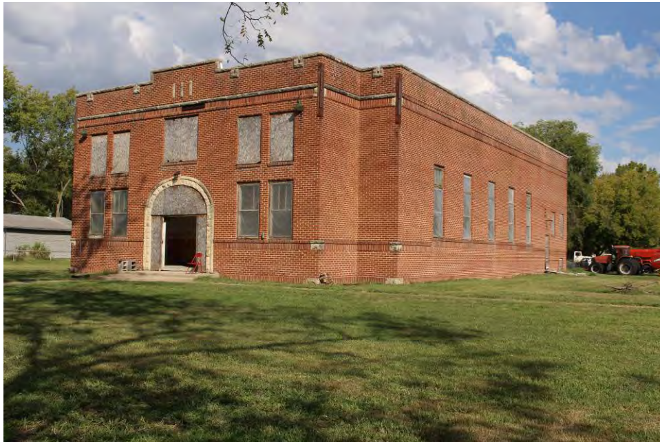
Photo 2: South (main) and east elevations
